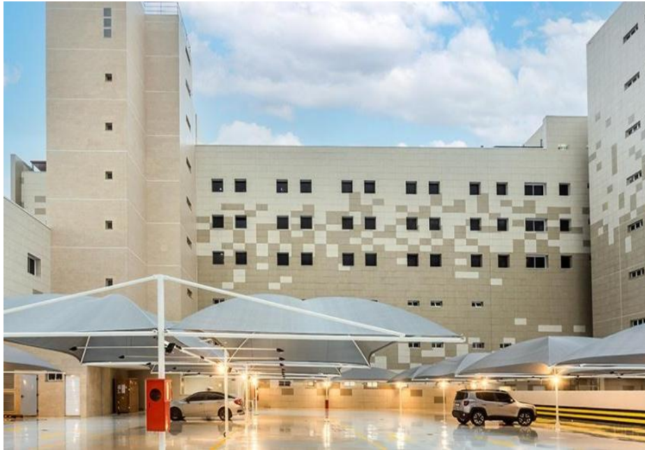
Figura 15: Fachada Ventilada do Hospital UNIMED PRIME
